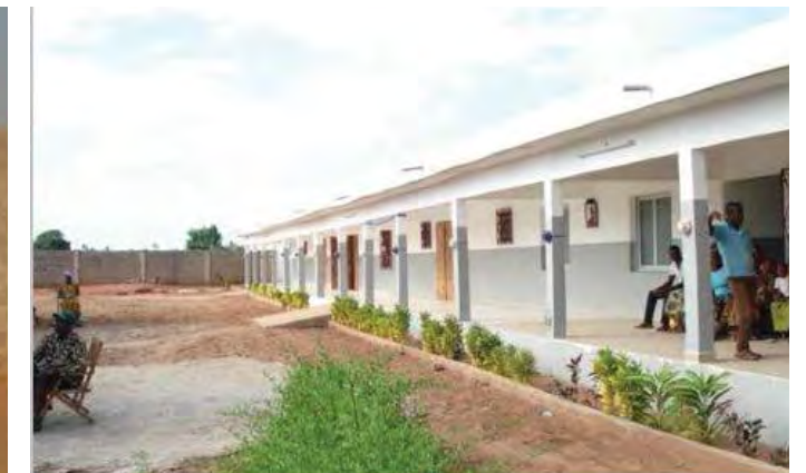
April 2014: The Centre de Secours Medical Fernando Giardinetti is ready to start clinical activity.
